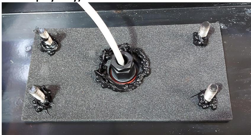
The sealant should be applied around the central hole (at approx. 60mm diameter) and directly around fixing studs to completely fill any gap between the stud and display gasket top face (See image above).
